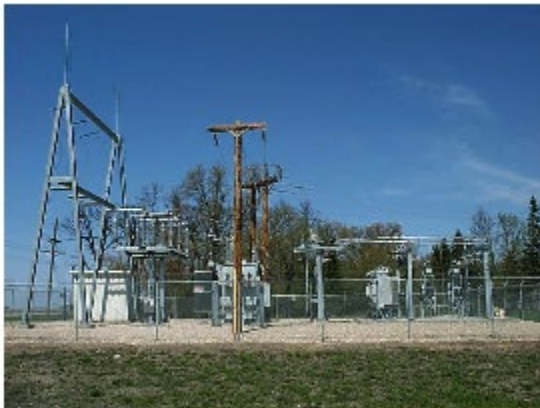
Image: Electrical substation
