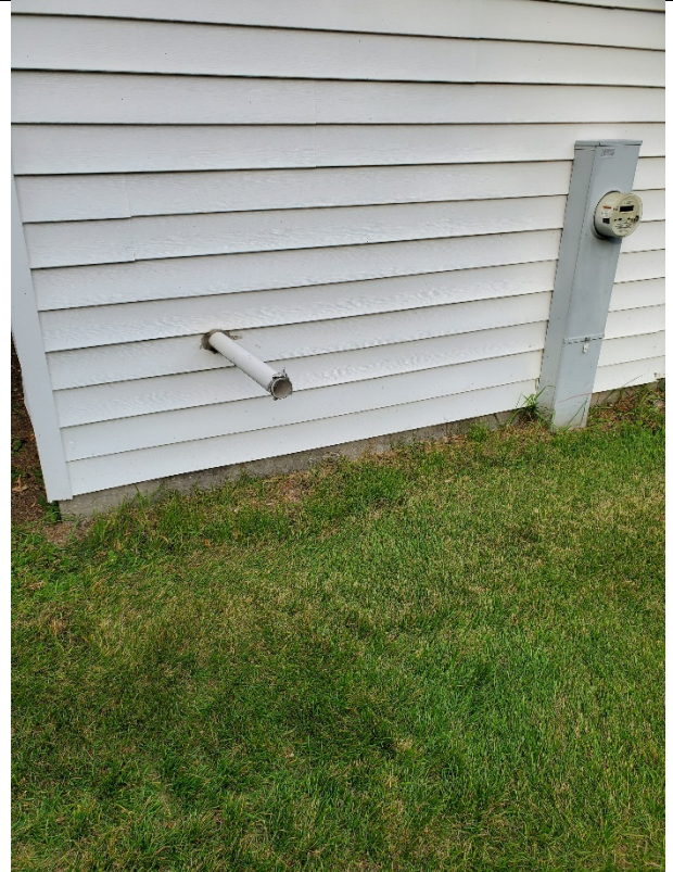
Photo 14: Screened discharge point from sump pump pit. Only about 18 inches from side of wellhouse when it should be at least 25 feet.
