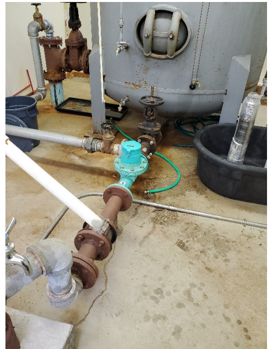
Photo 4: Check valve, water meter, 1,500 gallon storage tank and storage tank bypass line (going left)
