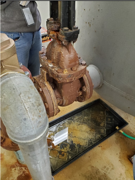
Photo 7: Leaking gate valve with visible corrosion.
