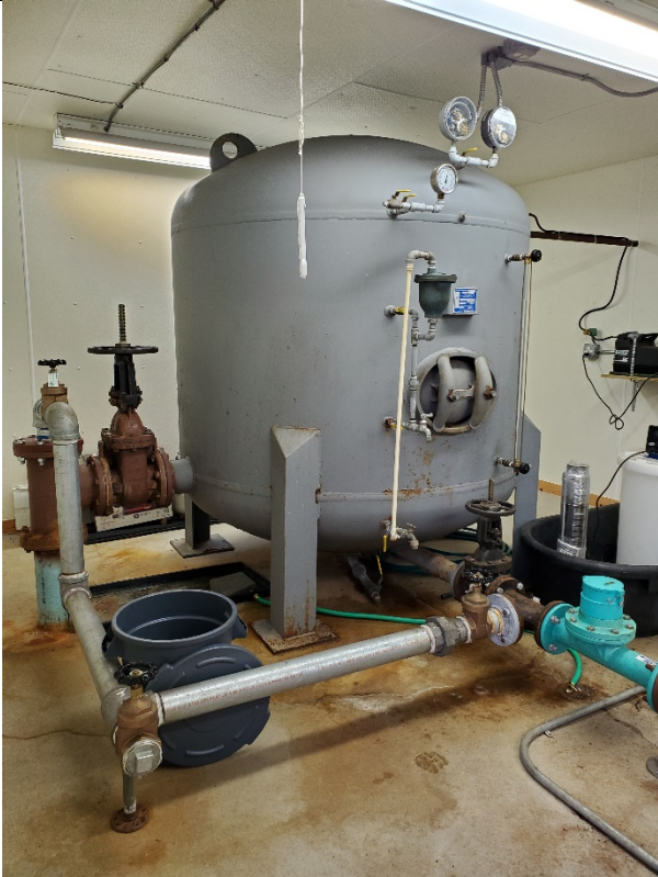
Photo 5: Steel storage tank in wellhouse, entry point sample tap, storage tank bypass line, outlet to distribution system (left)
