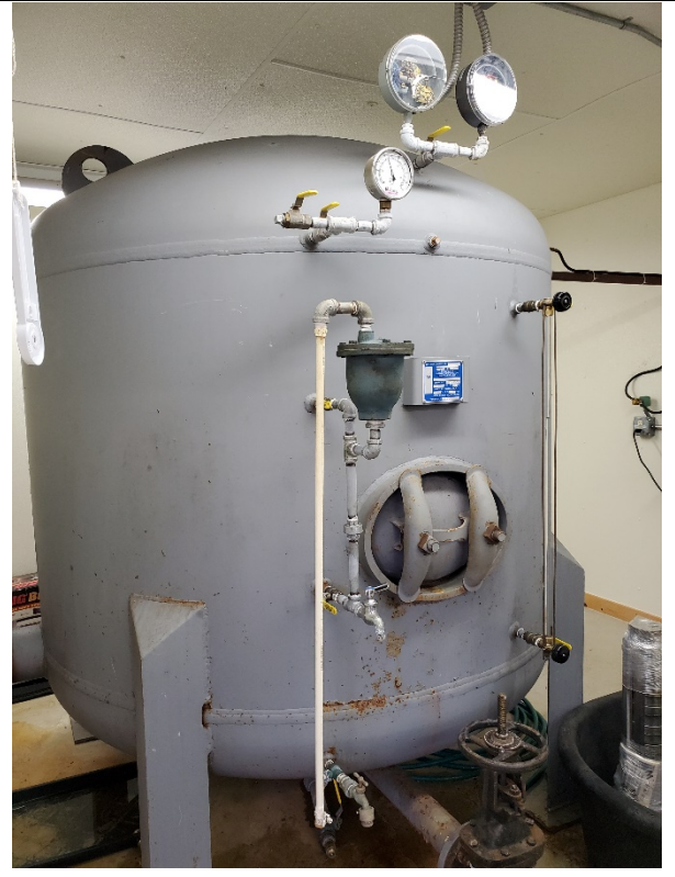
Photo 6: Entry point sample tap (center)
