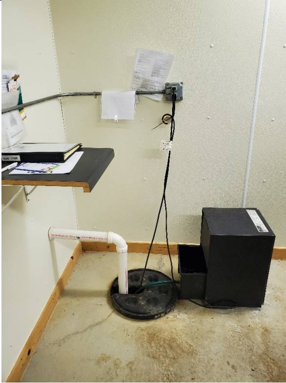
Photo 13: Wellhouse floor drain leads to sump pump pit. Dehumidifier drains here. Waste water is pumped through south wall of wellhouse.
