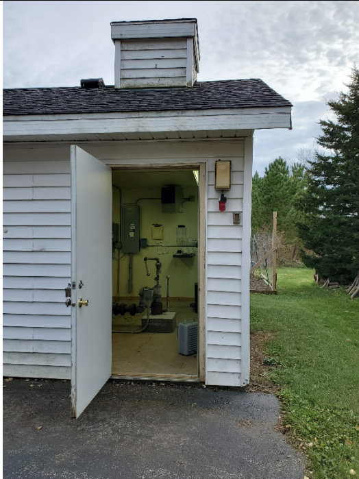
Photo 1: Wellhouse with outward opening door.
