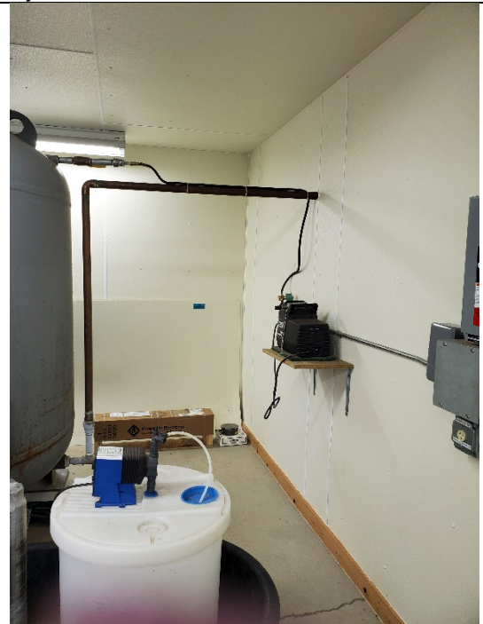
Photo 12: Screened line to exterior of well house.
