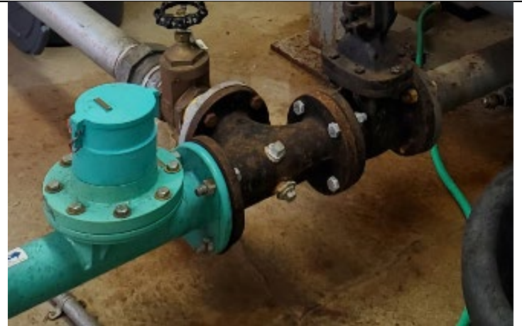
Photo 6: Entry point sample tap (center)
