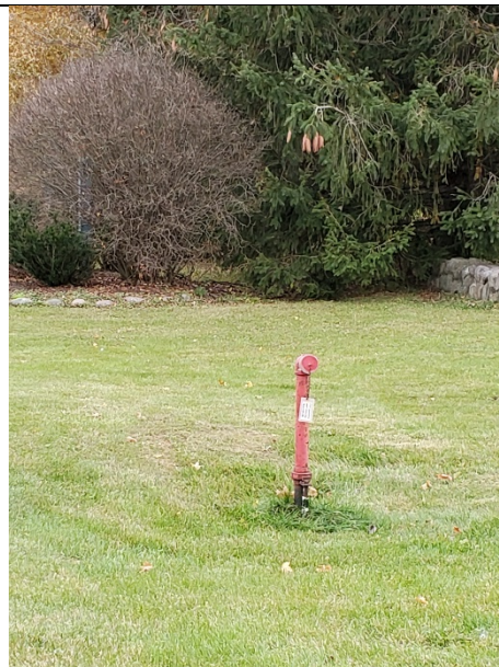
Photo 14: Screened discharge point from sump pump pit. Only about 18 inches from side of wellhouse when it should be at least 25 feet.
