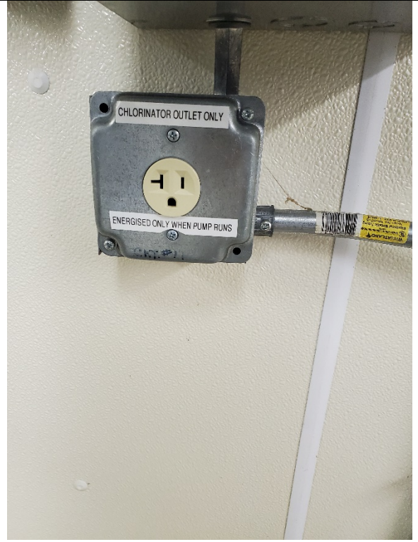
Photo 10: Dedicated electrical outlet for emergency chlorine system
