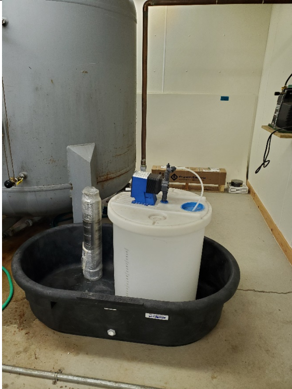
Photo 9: Emergency sodium hypochlorite injection system and spare submersible pump placed within spill containment.
