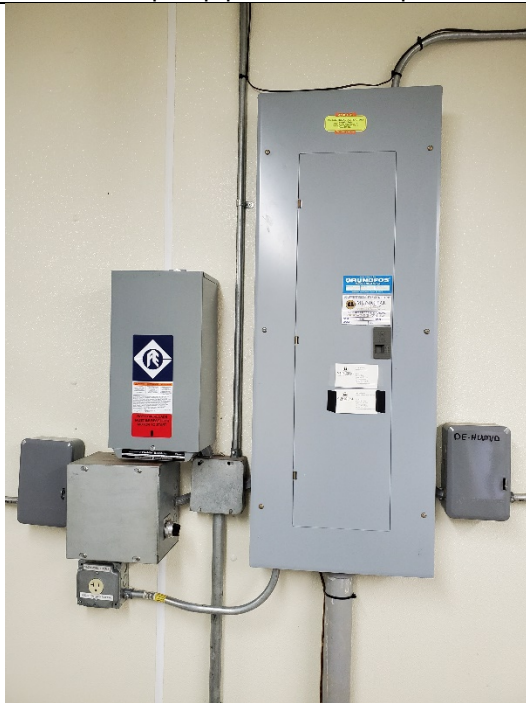
Photo 11: Pump control panel.
